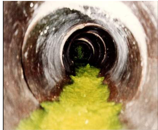
FIGURE 1.3.4 VIEW INSIDE SEWER PIPE FOR DYE TESTING
