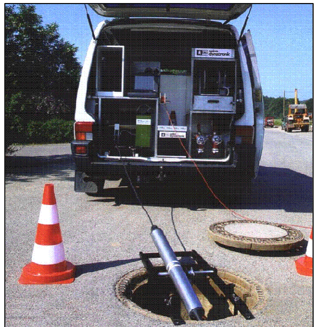
FIGURE 1.3.6 FOCUSED ELECTRODE LEAK LOCATOR SONDE AND EQUIPMENT VEHICLE FOR PIPE INSPECTIONS
