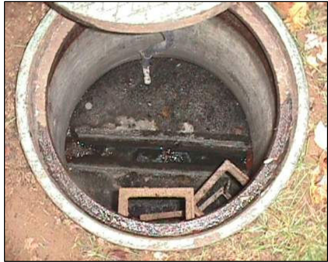
FIGURE 1.3.2 VIEW INSIDE A MANHOLE
