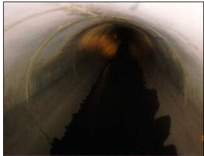
FIGURE 1.3.3 VIEW INSIDE SEWER PIPE FROM A TELEVISION INSPECTION
