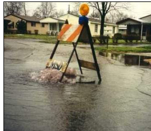
FIGURE 1.3.5 OVERFLOW DURING WET WEATHER
