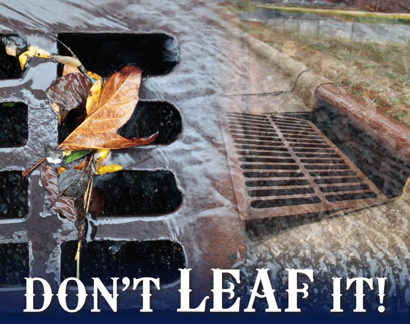
Catch basins carry stormwater away from our homes and streets when it rains. Covered or clogged catch basin drains, grates, and ditch lines contribute to street and yard flooding.
