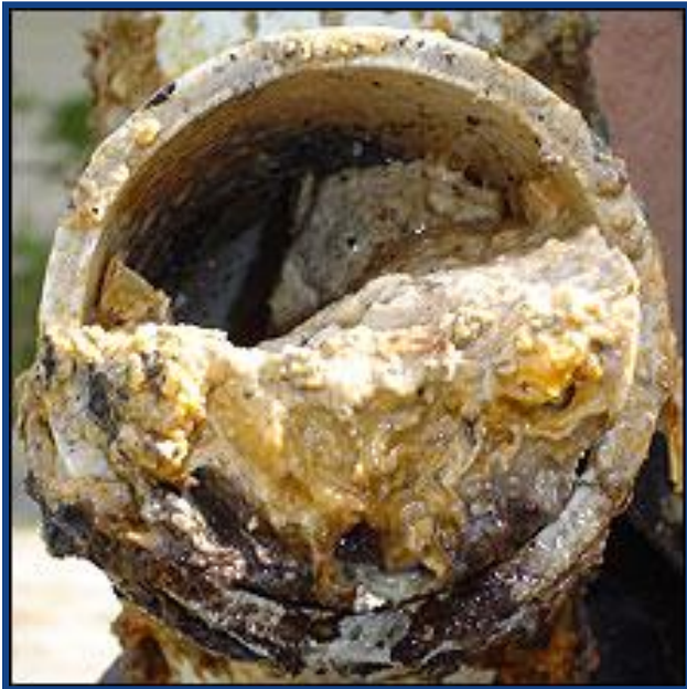
Grease accumulates in pipes
