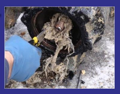
accumulates at pumps and causes sewer overflows and basement backups
