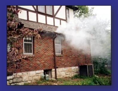
Smoke testing on public sewer indicates improper downspout connection to the sanitary sewer
