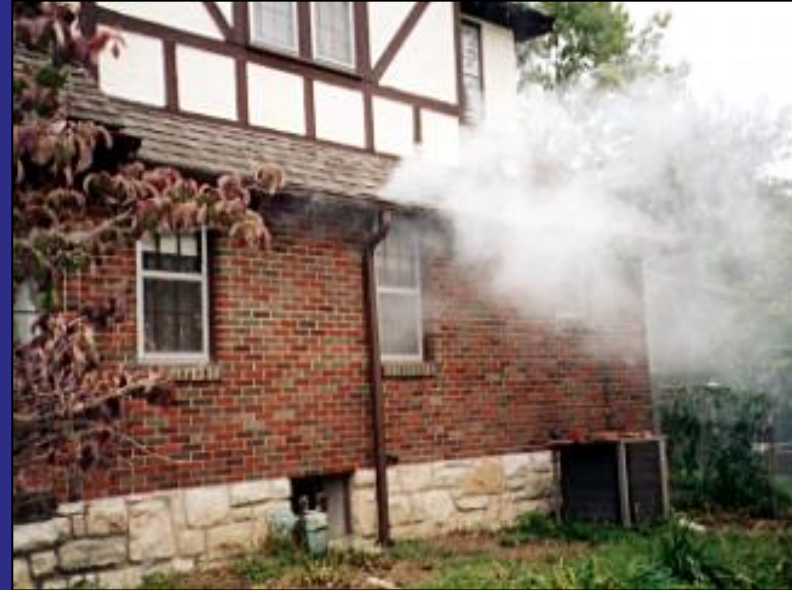
Smoke testing on public sewer indicates improper downspout connection
