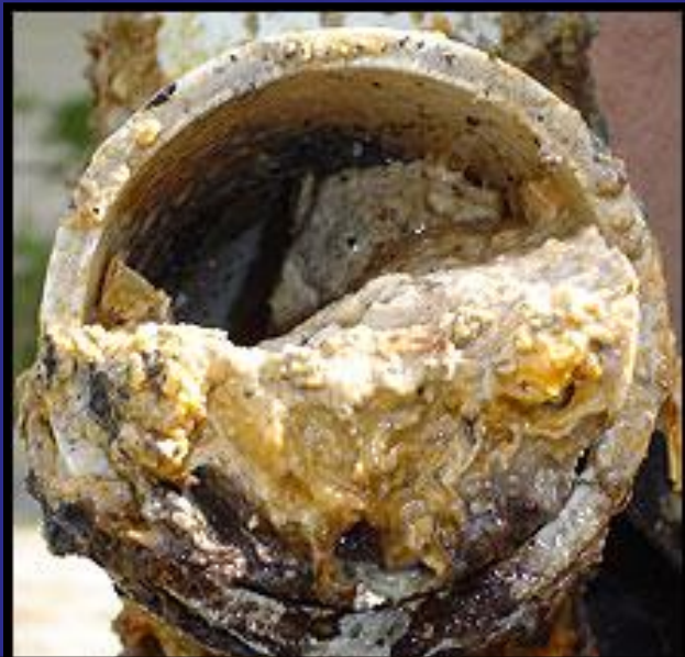
Grease accumulates in pipes
