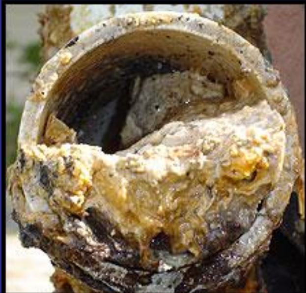
Grease accumulates in pipes
