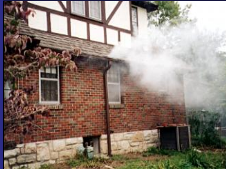
Smoke testing on public sewer indicates downspout connection
