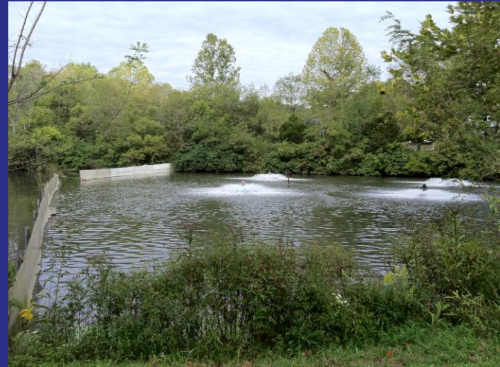
Lake of the Woods Sewage Lagoon
