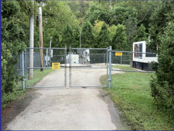
Chenoweth Run Pump Station
