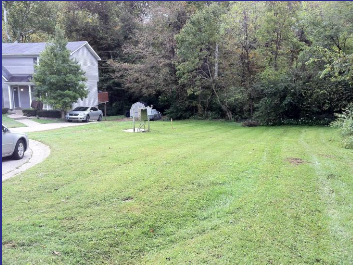
Lake of the Woods Lift Station
