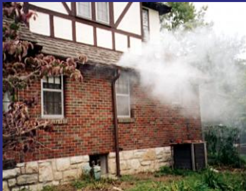
Smoke Testing for Illicit Connections
