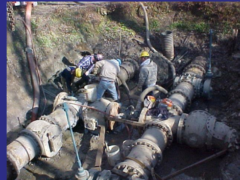
New Pipeline Construction
