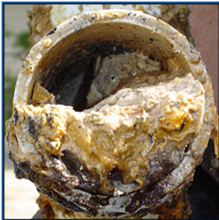
Grease accumulates in pipes
