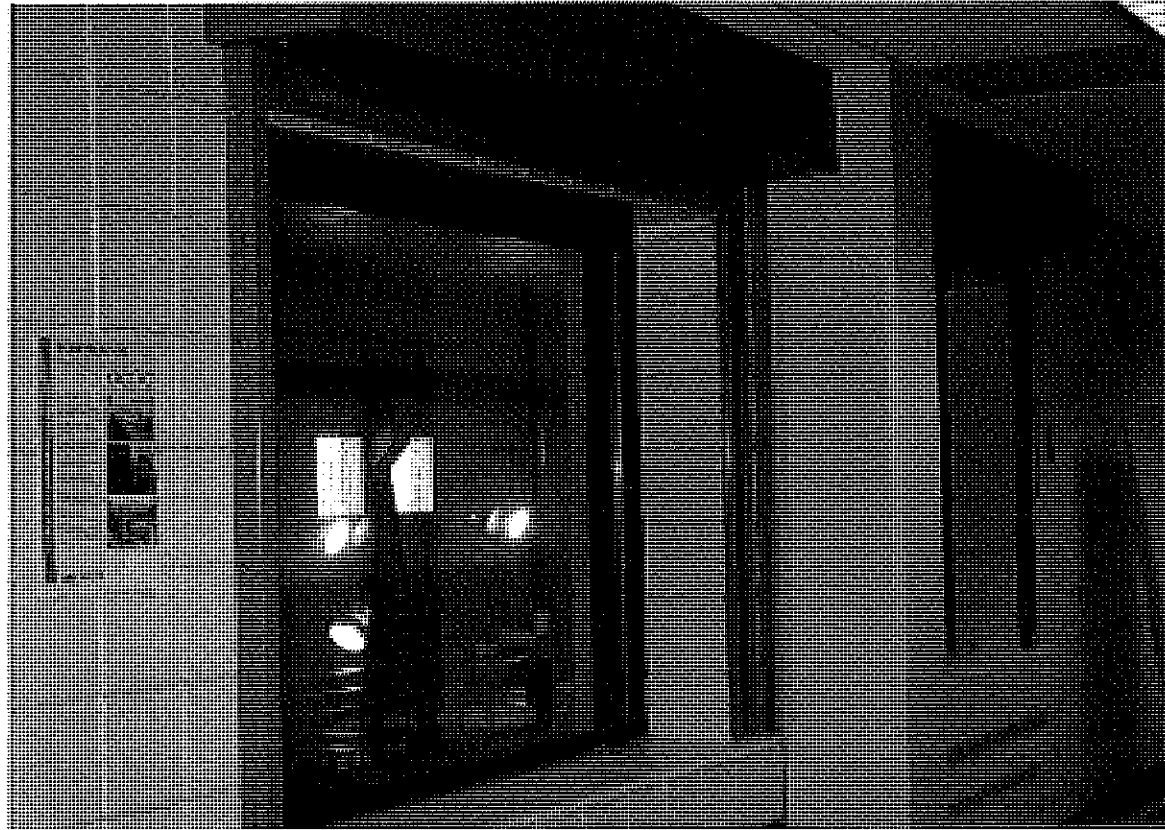
606 - GAK observation windows protected with drop-down panels
