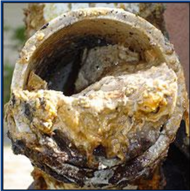
Grease accumulates in pipes
