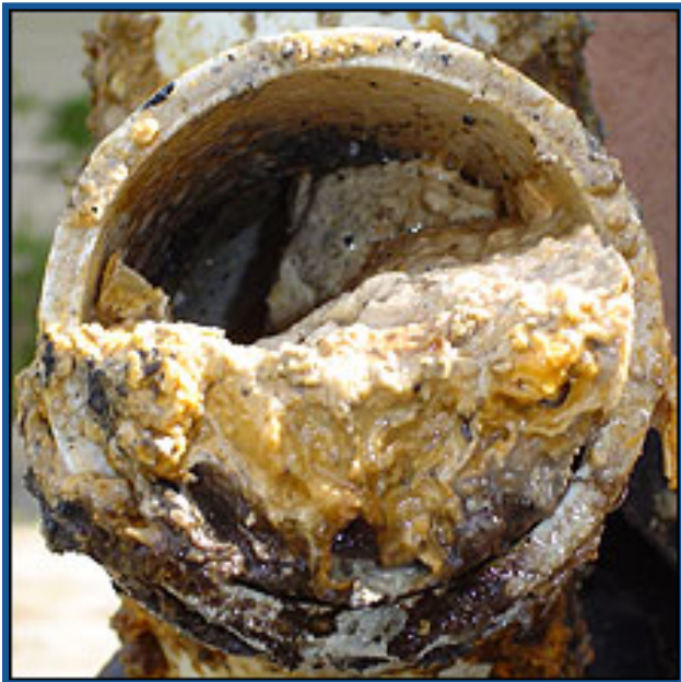
Grease accumulates in pipes
