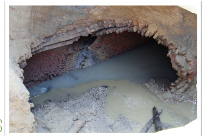
Broadway Sewer cave-in (originally built in 1867)
