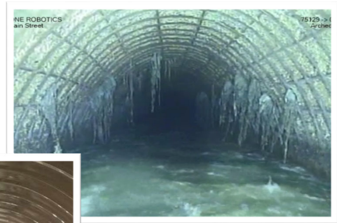
Ohio River Interceptor (West Main Street): Concrete deterioration and exposed rebar due to corrosion from sewer gases
