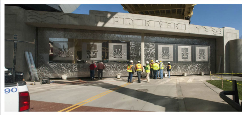
2nd and River Road Flood Gate
