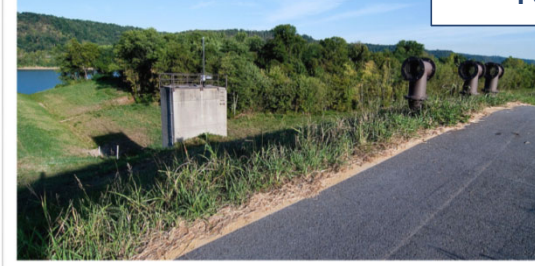
Floodwall Trail – SW Louisville
