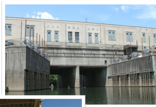
Beargrass Flood Pump Station
