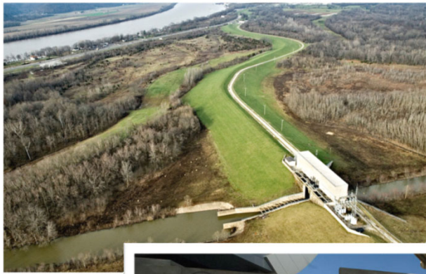
Pond Creek Flood Pump Station
