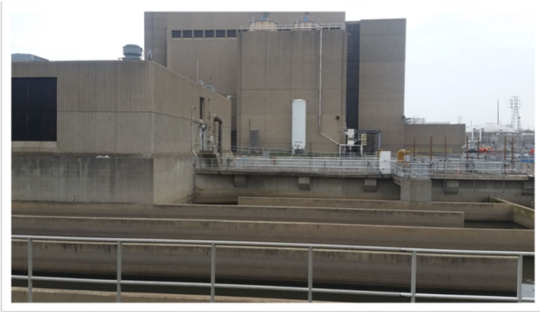
Morris Forman CSO Treatment Plant during Normal Operation
