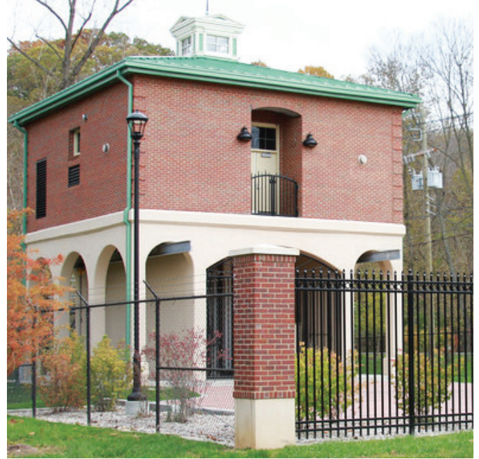
Mellwood Avenue Pumping Station
