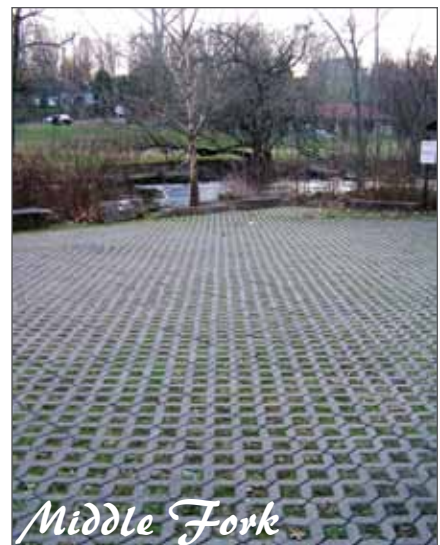
Pervious pavement reduces direct stormwater runoff to streams.
