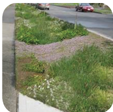
RAIN GARDENS and Bio-swales are shallow areas with amended soil that absorb rainwater runoff into the ground.
