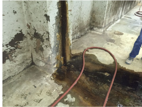
FIGURE 6-9 Leaking Expansion Joint
