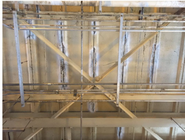
FIGURE 6-10 Damaged Concrete Roof Panels
