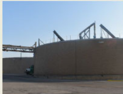
Limited Digester Capacity for Waste Activated Sludge
