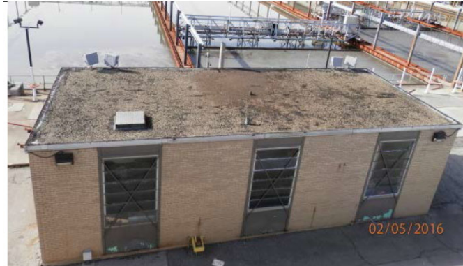
Built-up Roof on South Primary Pump Station
