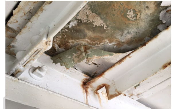
FIGURE 6-5 Corrosion on Steel Roof Framing
