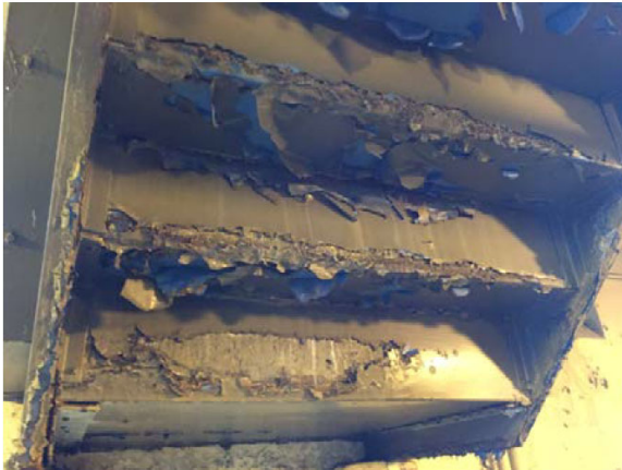
FIGURE 6-2 Corrosion of North Staircase
