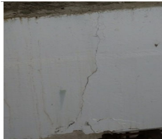
FIGURE 6-9 Leaking Expansion Joint
