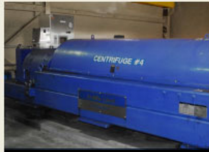
Typically 3 of 5 Dewatering Centrifuges in Operation– Not Keeping Up with Demand
