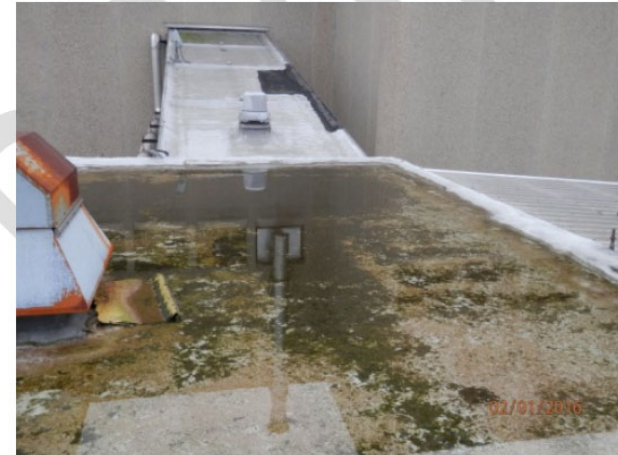
Ponding water with debris approximately \frac{3}{4} inch in thickness.
