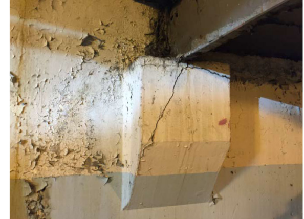
FIGURE 6-3 Cracked Concrete Haunch
