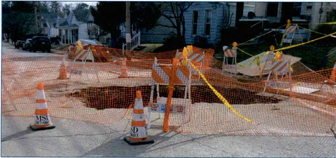
Schiller Ave sewer collapse, January 2016 Originally built in 1912
