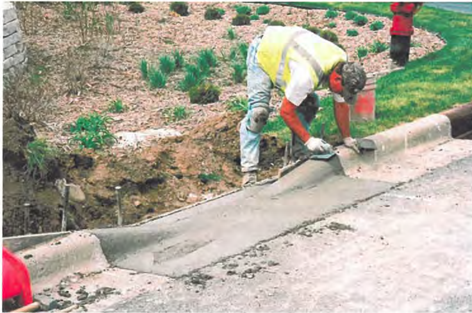
Cuts in the curb allow stormwater to enter the gardens from the street.
