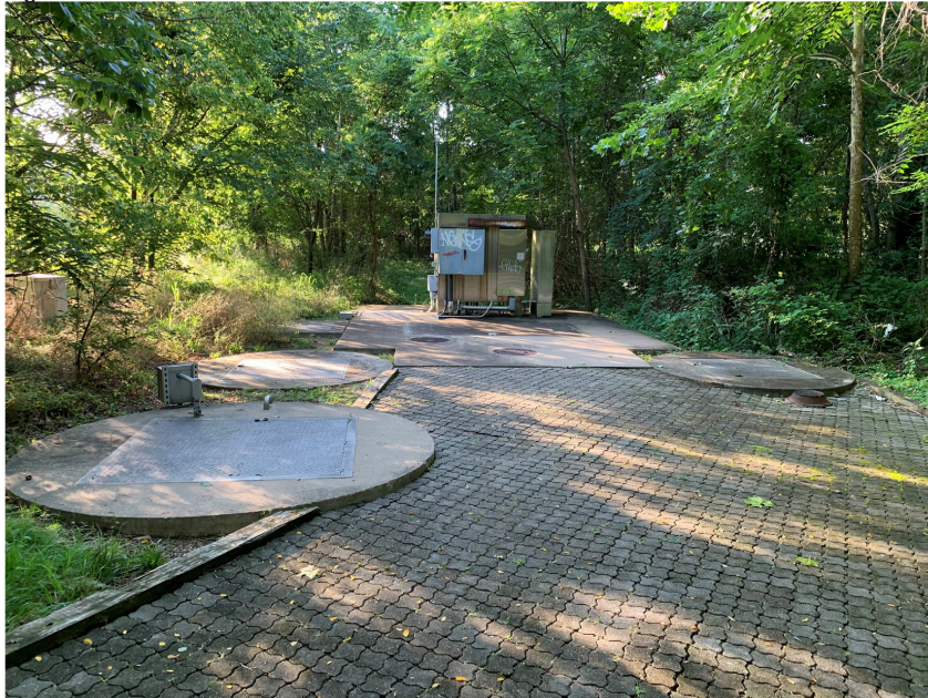
Figure 2. Entrance to CDS Unit
