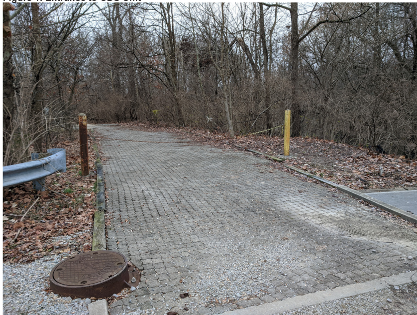
Figure 1. Entrance to CDS Unit
