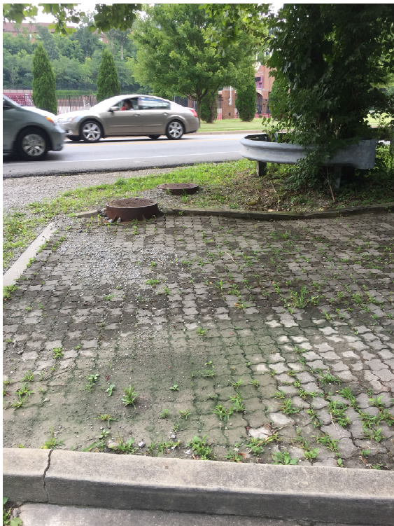
Figure 2. Entrance to CDS Unit
