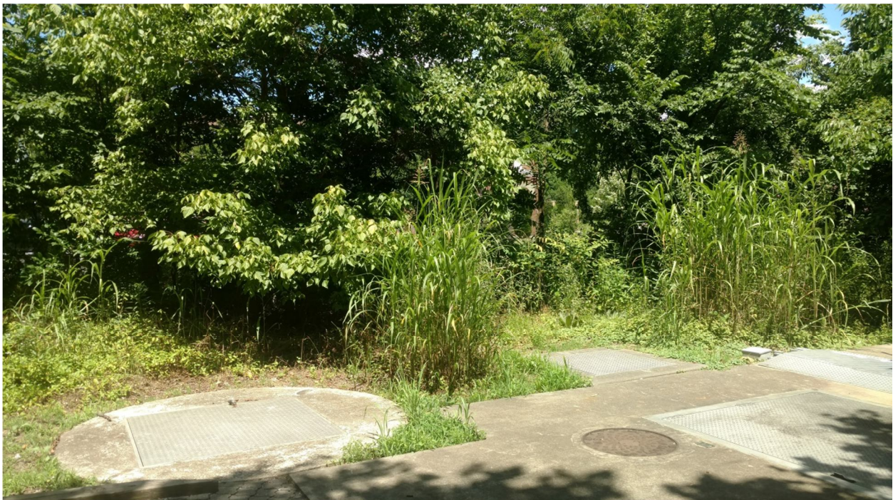
Figure 4. Area Adjacent to the CDS Unit
