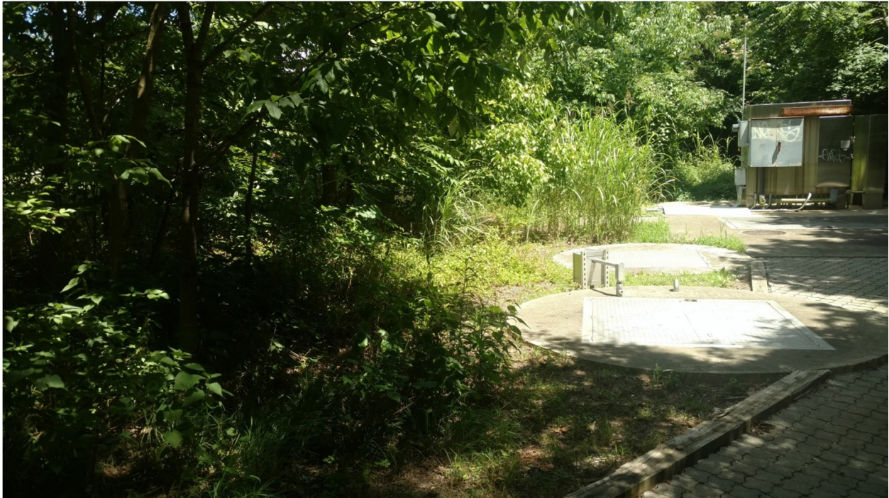
Figure 3. Area Adjacent to the CDS Unit
