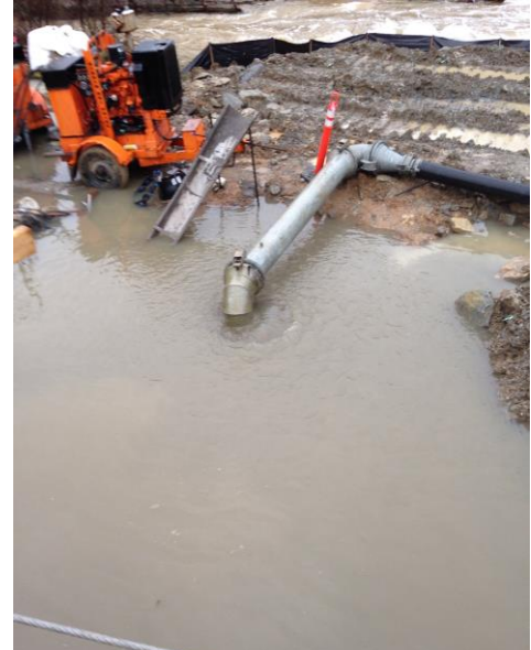
Fairmount Road Storage Basin De-Watering Line & Overflow at Manhole 116106.
