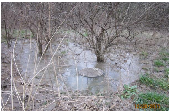
Manhole 97365 in field across street from Fairmount Road
