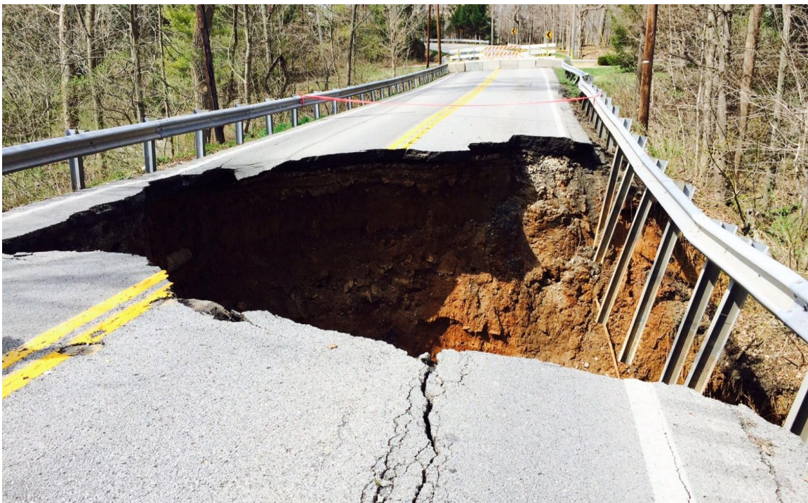
KY 22 washed out by floods April 3, 2015. National Weather Service Photo: http://www.weather.gov/lmk/april_2015_summary
