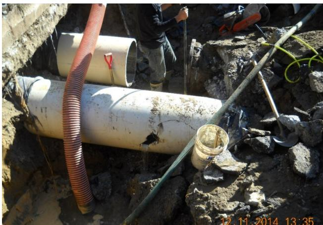
Excavation showing break in south barrel of ORFM.
