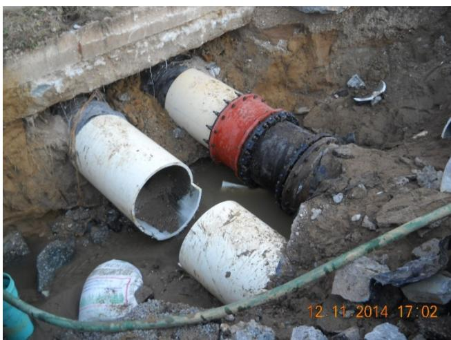
Excavation showing north barrel of ORFM repaired.
