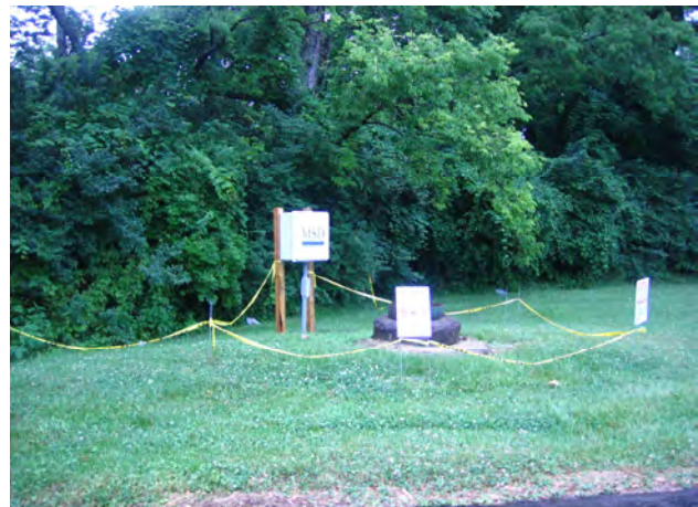
Control Zone Materials – Manhole 28173
