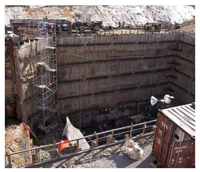
completed and two new clarifiers being excavated and concrete pours initiated during this period. Excavation on the new chlorine basins contact and the new Grit Facility is also underway. Completed work has reached the 30% stage. On the PP, the Short Term Detention Basin walls have been poured and the footings for
