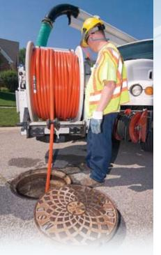
Above: Dan Bailey flushes and cleans a neighborhood sewer to prevent buildup of fats, oils and grease, which is shown in the photo below.
