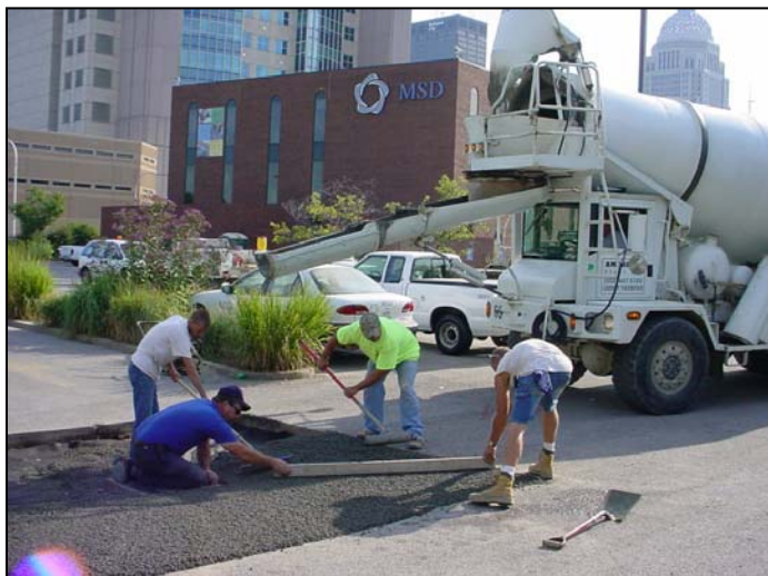
Installation of Pervious Concrete at the Main Office
