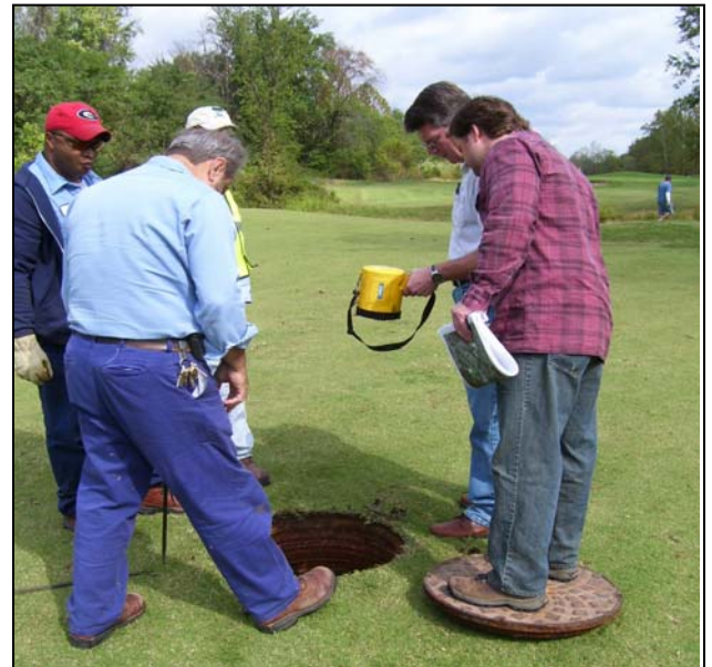
Crew locates a force main
