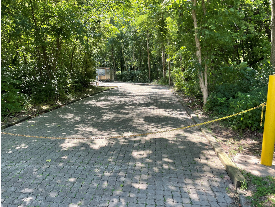
Figure 1. Entrance to CDS Unit
