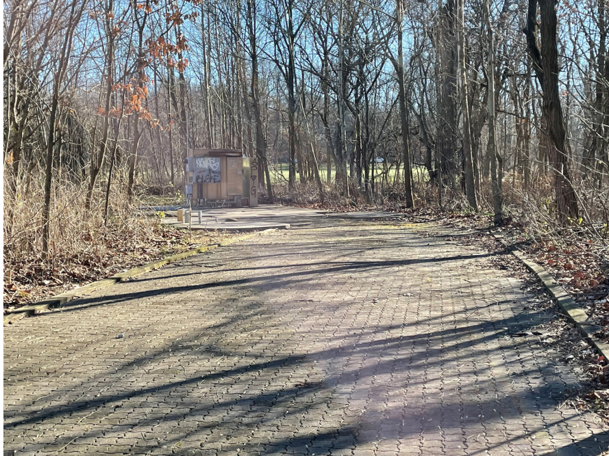
Figure 1. Entrance to CDS Unit
