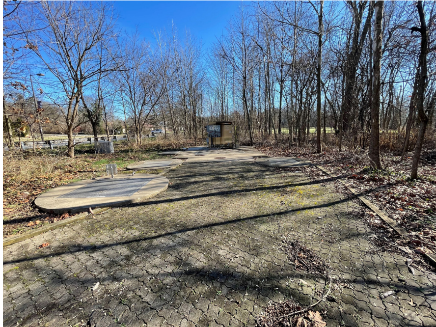
Figure 2. Entrance to CDS Unit
