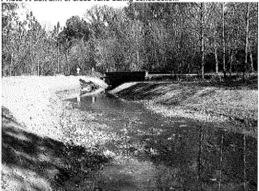
Photo 8: Riffle constructed using native gravel and J-hook directing flow through bridge opening.
