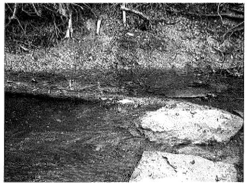
Photo 15: View of flow over log vane following construction
