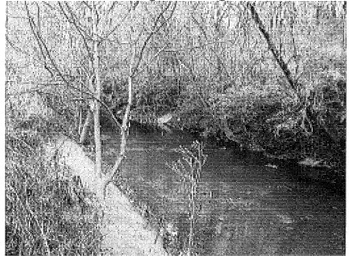
**Photo 16:** Left bank located downstream of project treated with live brush layering and soil wraps protected with coir fiber matting. This area was added to the project through a change order.
