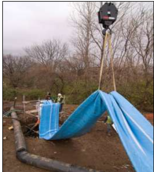
Figure 5 - Cast in place pipe is installed to rehabilitate long stretches of dilapidated sewer mains
