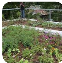
GREEN ROOFS capture stormwater with vegetation or other devices before it drains into sewers and waterways.
