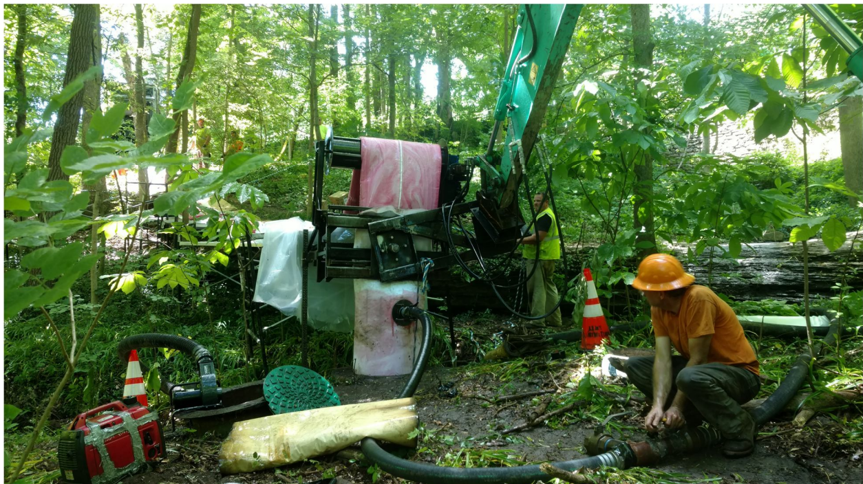
Figure 2-3 Cured-In-Place Pipe (CIPP) Installation
