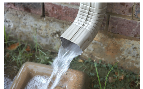
This downspout is not connected to the sewer system.
