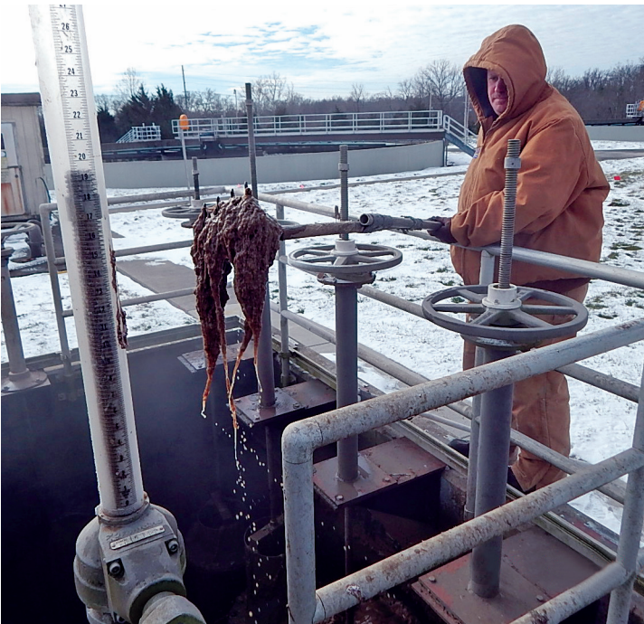
Shawn Smith clears a clog from a pump at MSD's Cedar Creek Water Quality Treatment Center.
