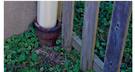
Downspouts connected to the sewer system, such as the one shown above, can overwhelm the system and contribute to sewer overflows.
