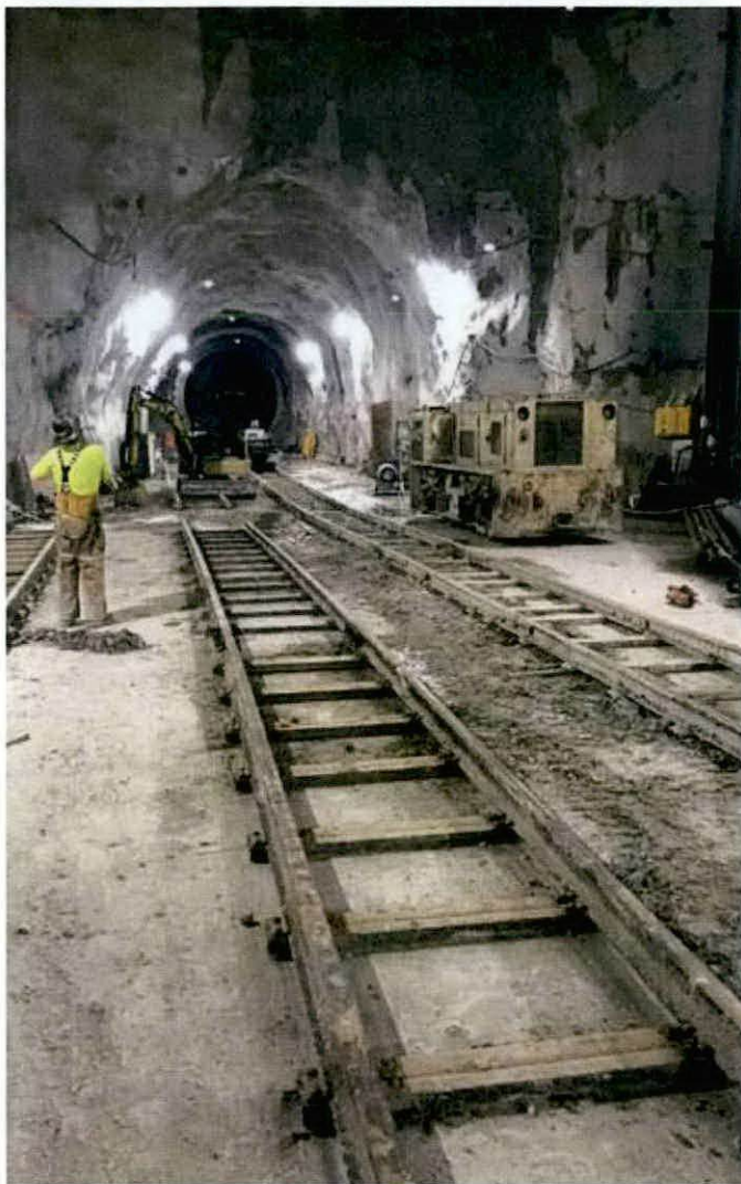
Crews work to install a rail line to transport both workers and rock through the tunnel.
