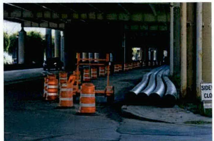
Pipes for the temporary pump-around are ready for installation along River Road.
