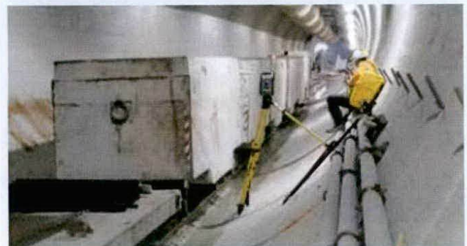
A crew member waits for the muck car train to pass before completing his survey. Muck cars move rock from the boring machine for transport out of the tunnel.
