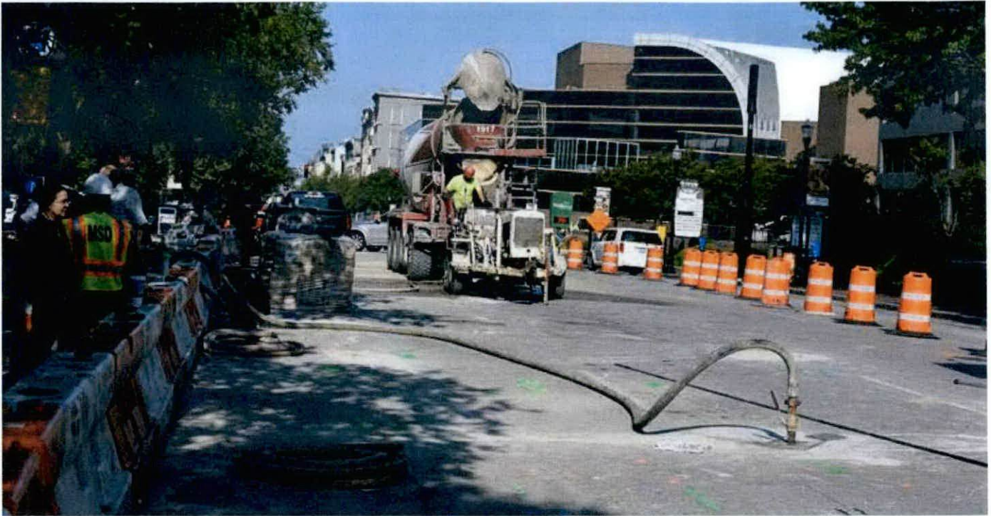
Contractors work to fill the void underneath the West Main Street pavement. A cave-in and heavy rains removed most of the supporting soil under this portion of the roadway.
