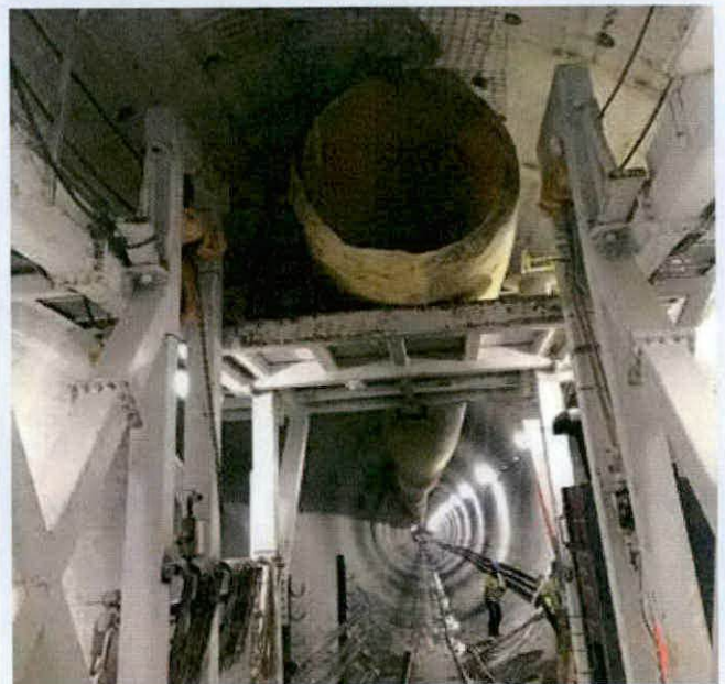
Ventilation shafts pump fresh air to workers who are 200 feet below ground.
