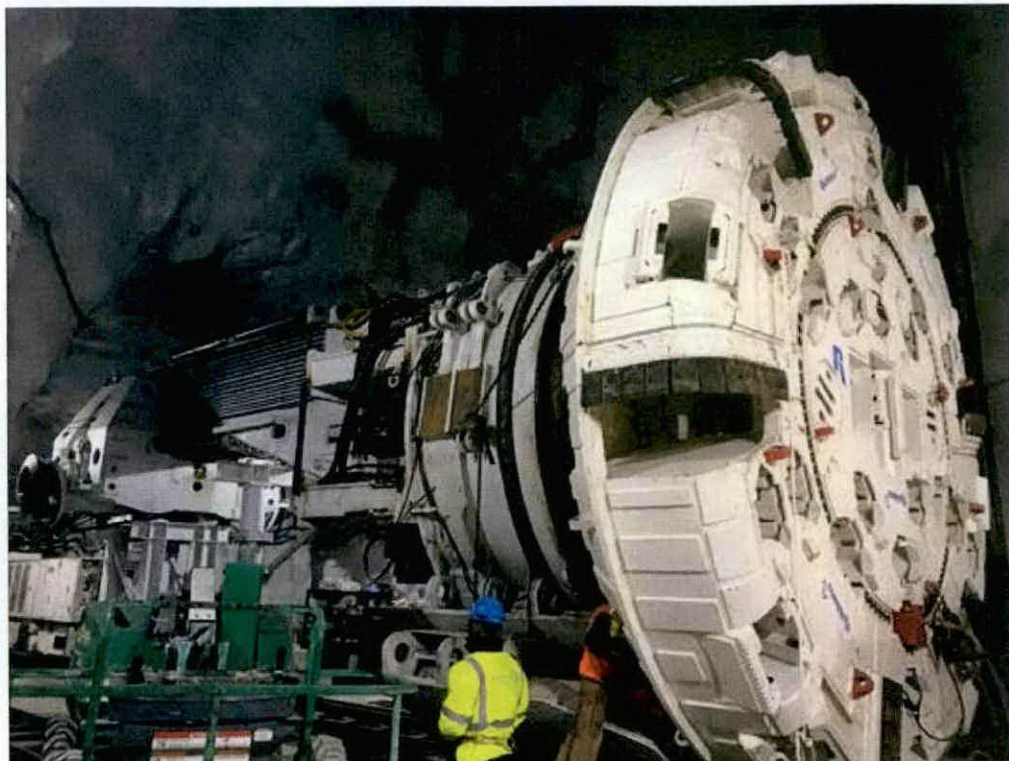
Assembly for Bumblebee's giant 22-foot diameter cutterhead proceeds underground in preparation for cutting through 4 miles of rock to form MSD's Waterway Protection Tunnel.
