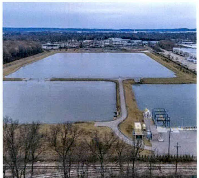
Buechel Basin is a series of storage areas that protect the community by holding a total of 104 million gallons of stormwater overflow, which is equal to a 10-year storm.
