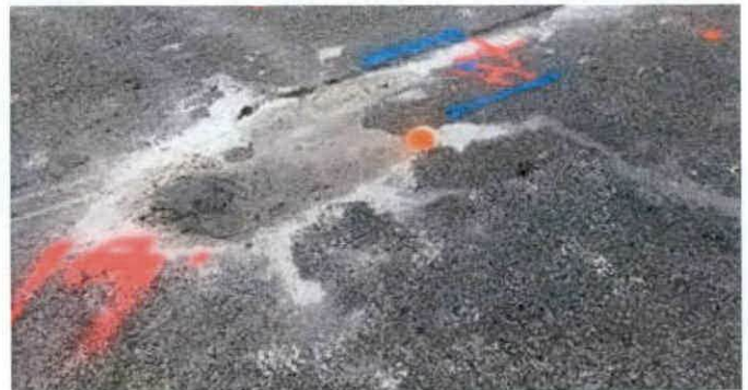
The pink "X" marks the spot of the cave-in of the West Main Street sewer 25 feet below. The pink "19" gives the depth of the void at that point under the pavement.
