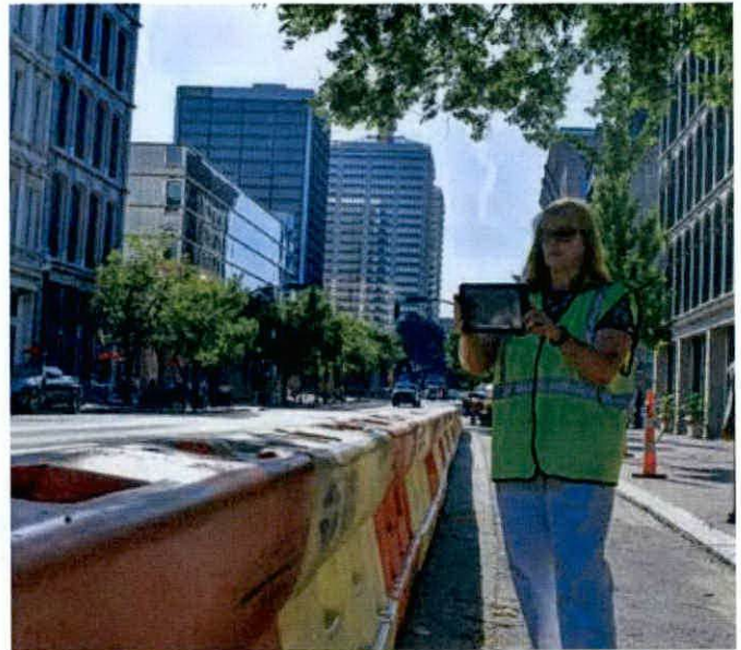
Inspectors regularly look for changes in the pavement that might indicate a cave-in.
