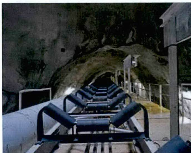
This conveyor system allows removal of the excavated rock as Bumblebee's cutterhead buzzes through 4 miles of rock.
