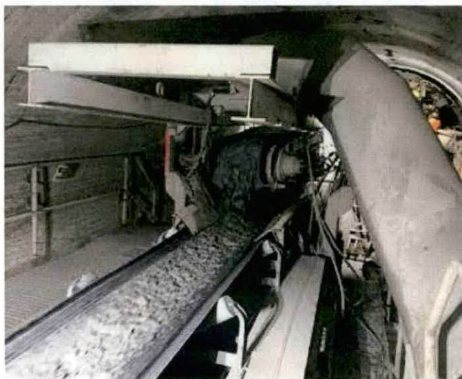
Excavated rock leaves the back of the boring machine by way of a conveyor belt. The rock travels to the tunnel's working shaft, where it is lifted out in muck cars by a crane.
