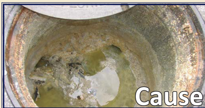
Grease Accumulating in Sewer Manhole
