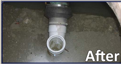
Same Grease Trap After Repairs and Cleaning
