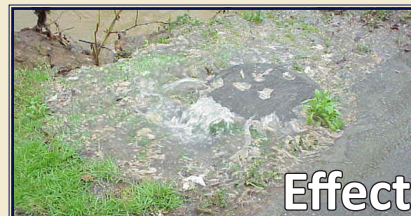
Sanitary Sewer Overflow Caused by Grease Accumulation
