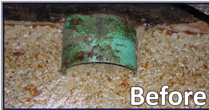
Poorly Maintained & Malfunctioning Grease Trap
