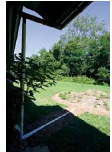
Water redirected from the roof gutter now flows into this Rain Garden at The Louisville Nature Center
